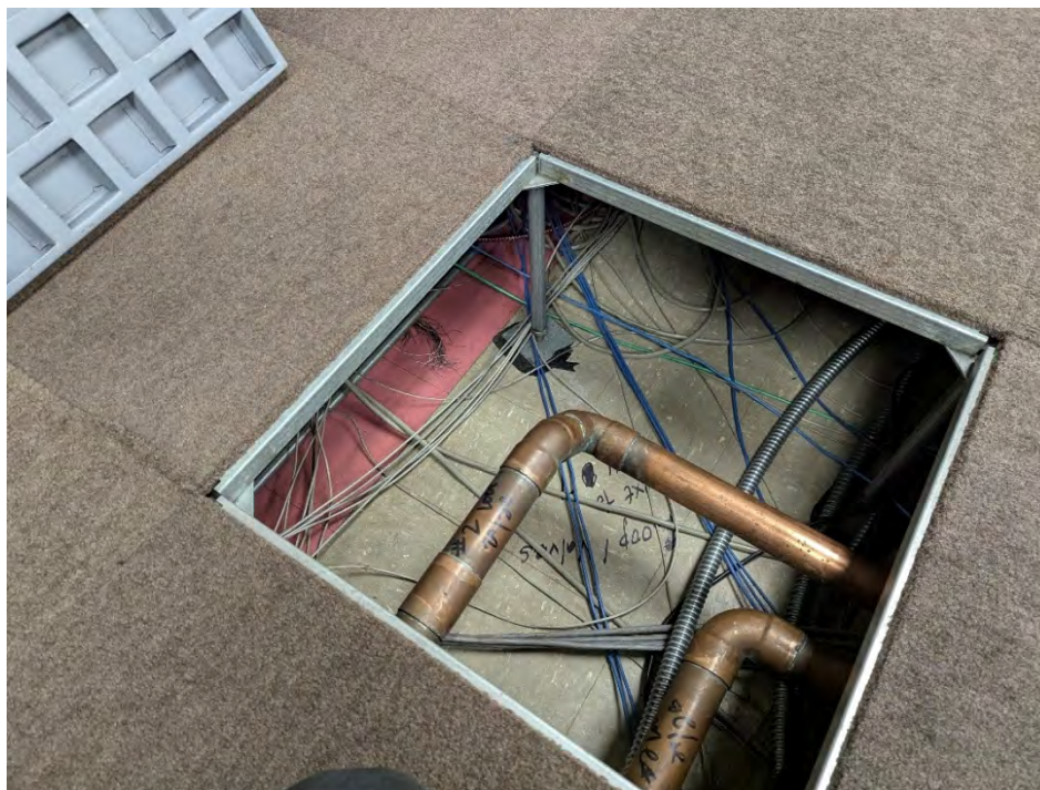
Photograph 6: Black mastic associated with red 12x12" floor tile, observed in the Addition. Sample number 66-B.
