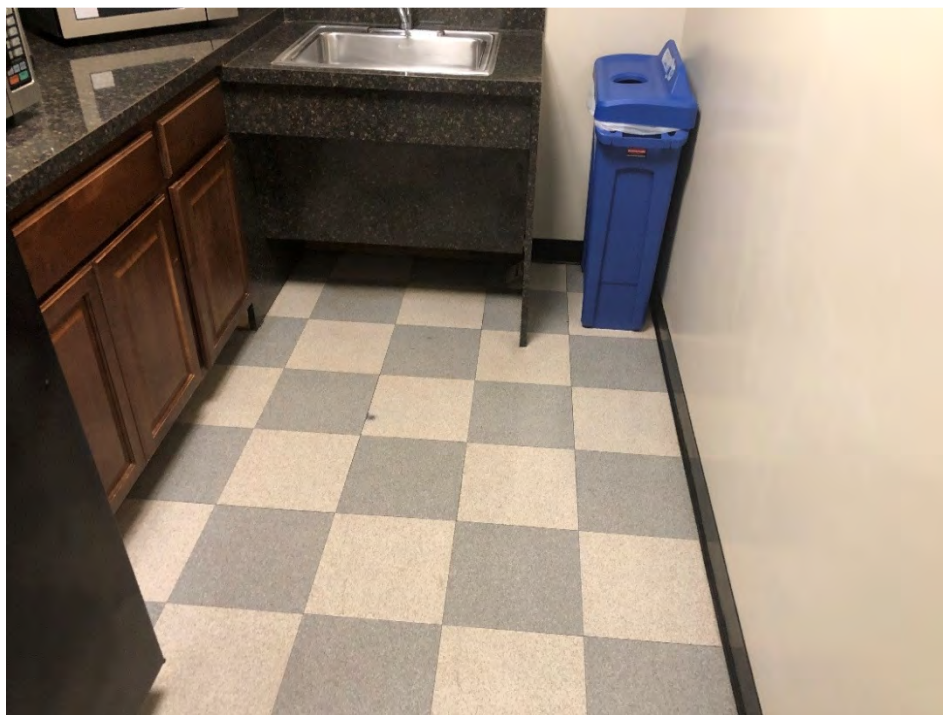
Photograph 7: Brown mastic associated with gray with black and white specs 12x12" floor tile and white with black and grey specs 12x12" floor tile, observed in the Tower. Sample numbers 61-B and 63-B.
