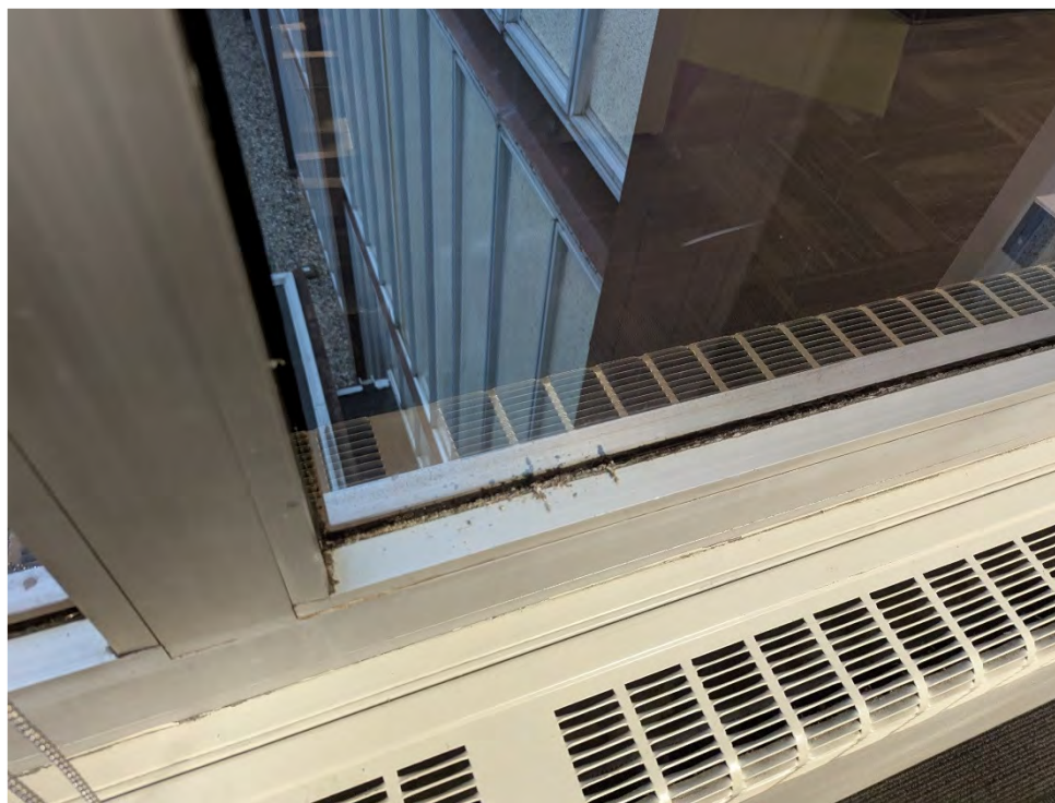
Photograph 12: Black interior window caulk, observed in the Addition. Sample number 26.
