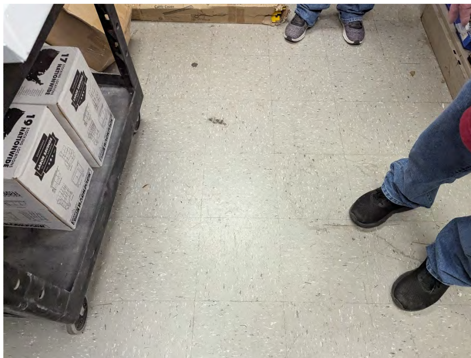
Photograph 2: Gray 12x12" floor tile, observed in the Original building. Sample number 68-A.
