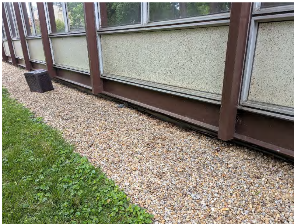
Photograph 17: Concrete waterproof sheeting, observed in the Addition and Tower. Sample numbers 119 and 118, respectively.
