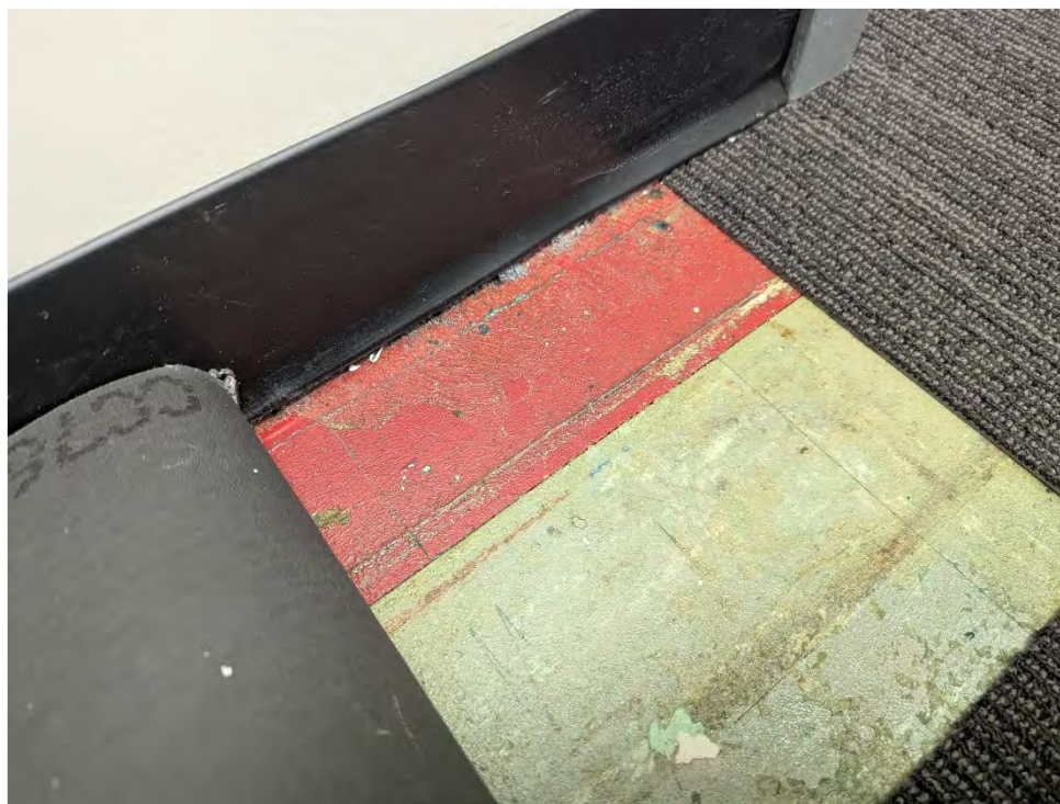
Photograph 4: Red 9x9" floor tile that has black mastic, observed in the Original building. Sample number 174-B.
