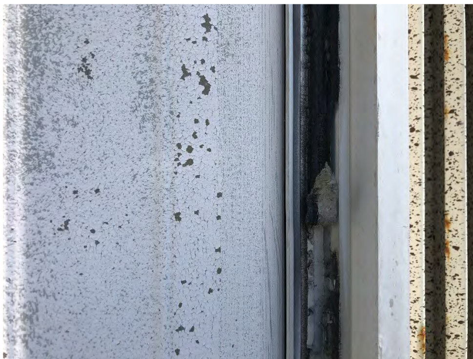
Photograph 14: Silver/gray sealant on exterior panel of mechanical wall, observed on the Addition. Sample number 107.
