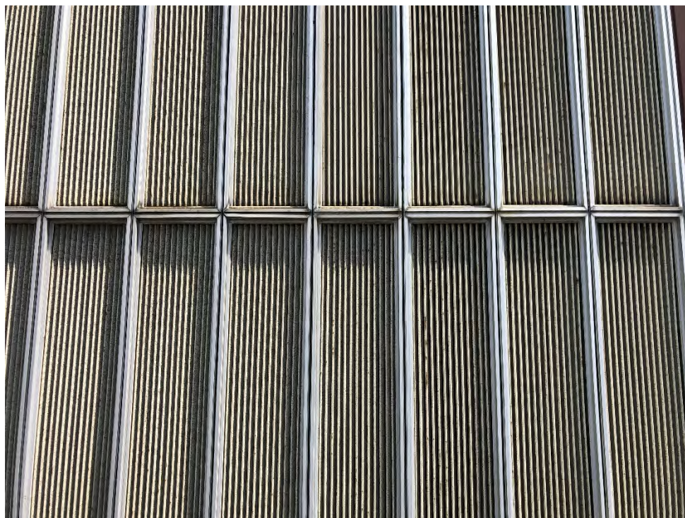
Photograph 15: Silver/gray sealant on exterior panel of mechanical wall, observed on the Addition. Sample number 107.
