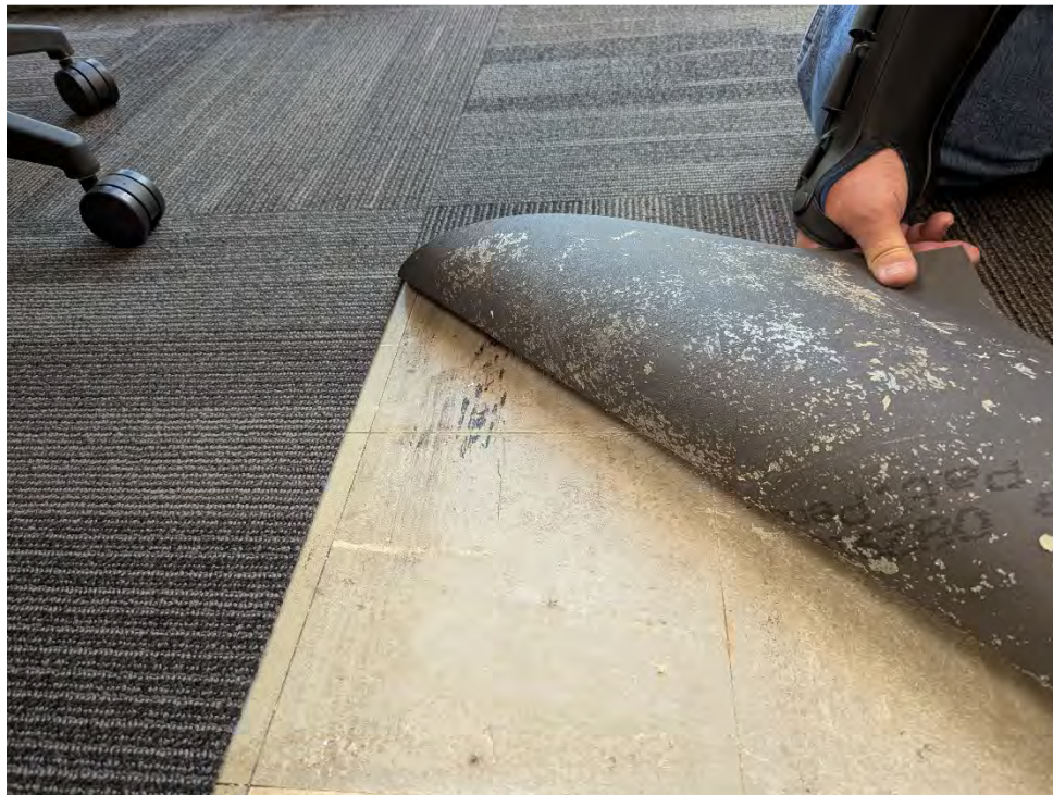
Photograph 1: Gray 9x9" floor tile, observed in each building. Sample numbers 62-B and C, 11-B and C, and 41-B and C.
