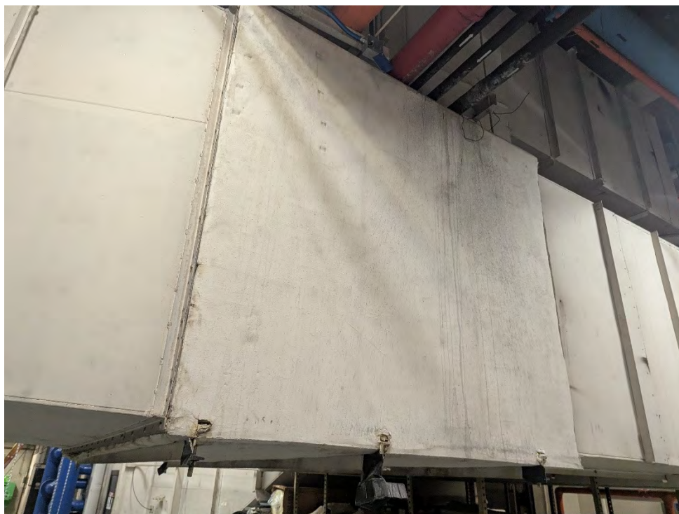
Photograph 20: Canvas on duct, observed in the Tower. Sample number 16.
