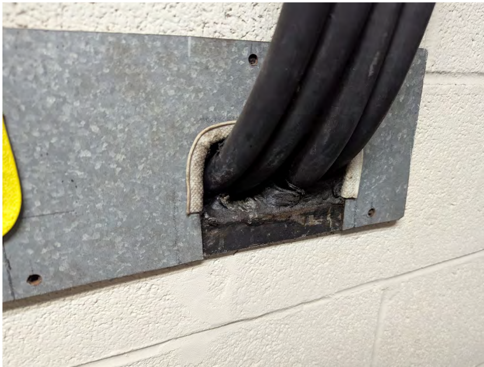
Photograph 13: Black penetration sealant, observed in the Addition. Sample number 79.
