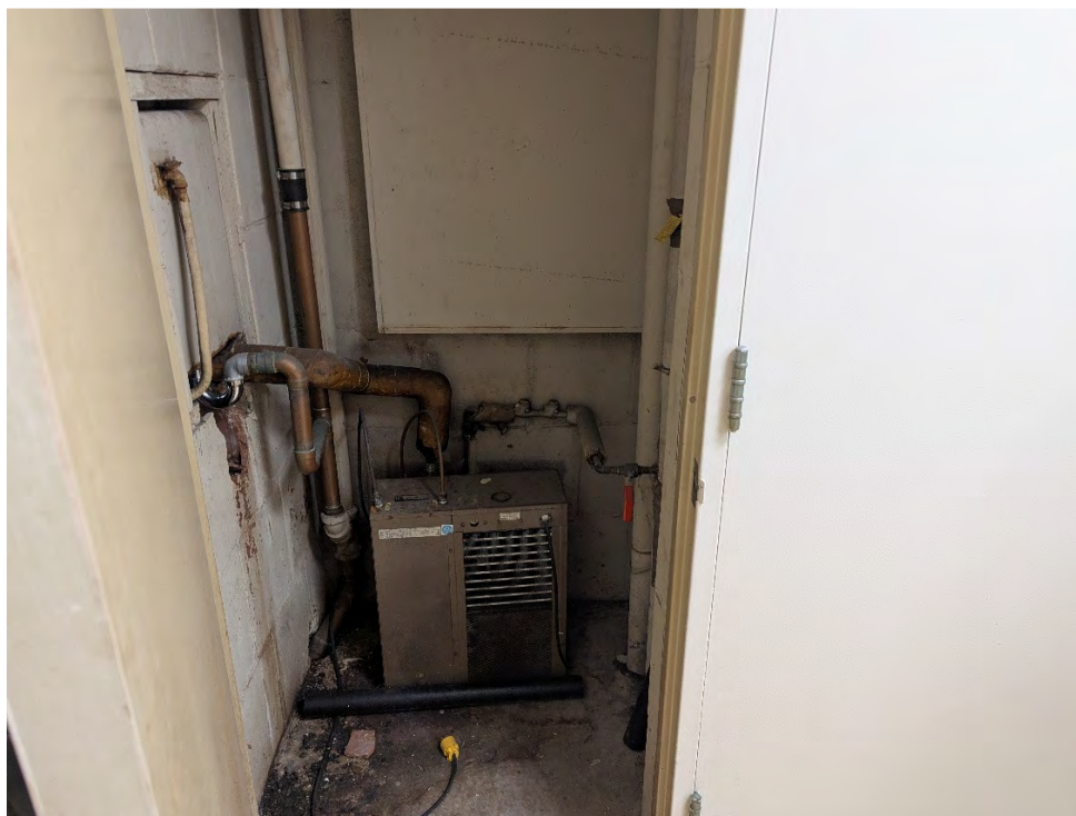
Photograph 24: 1"-3" pipe fitting, observed in the Original building. Sample number 149.
