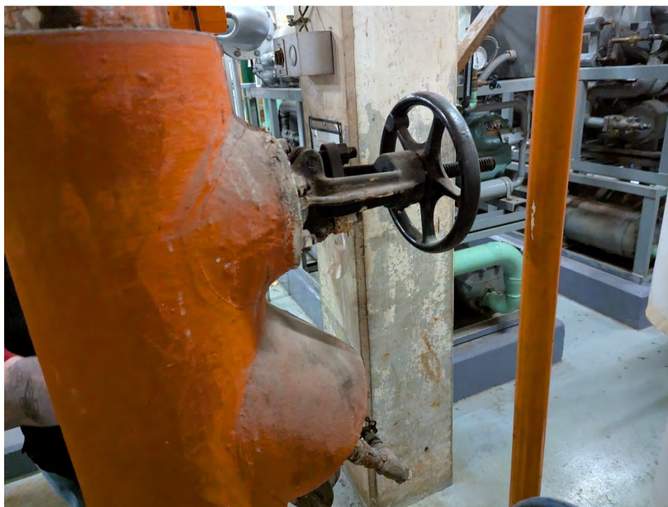
Photograph 23: 12" pipe fitting (orange), observed in the Original building. Sample number 106.
