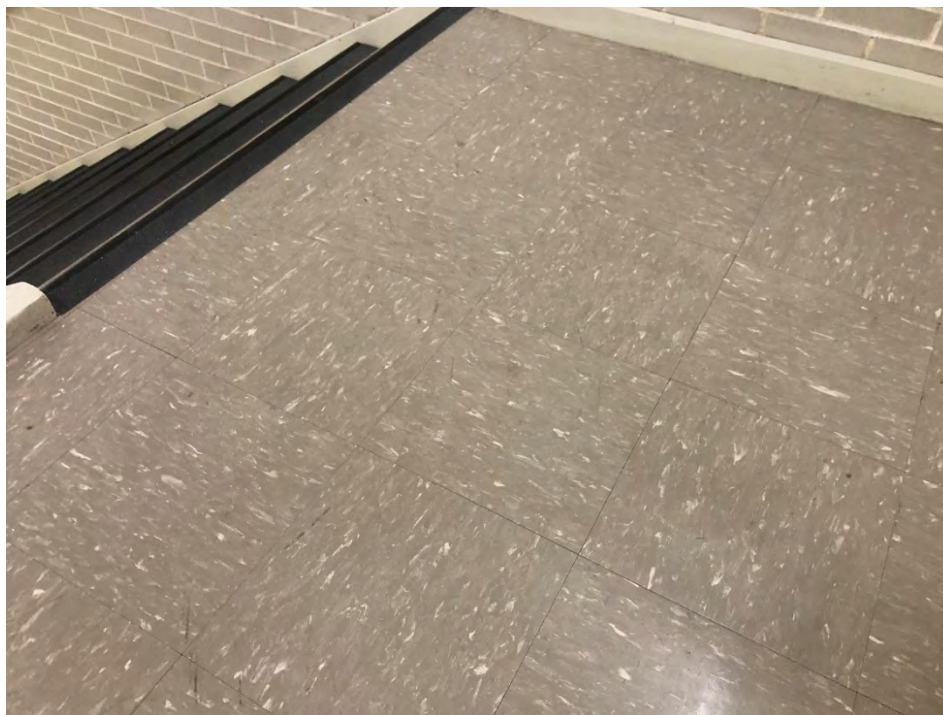
Photograph 8: Gray with white streaks 12x12" floor tile, observed in the Tower. Sample number 69-A
