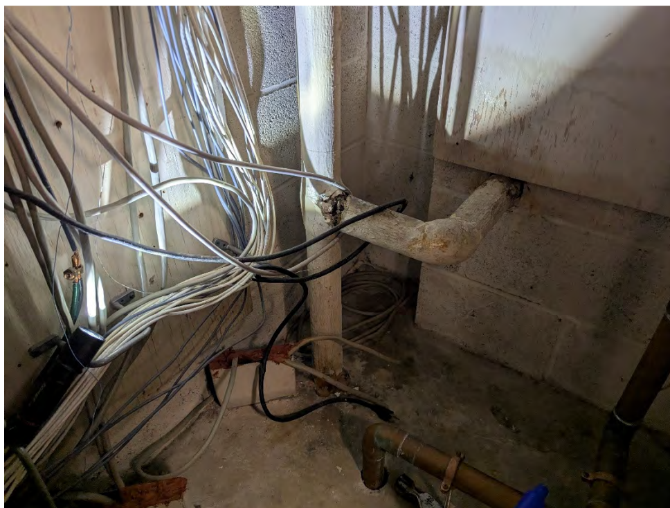
Photograph 27: 1"-3" pipe fitting, observed in the Addition. Sample number 19.
