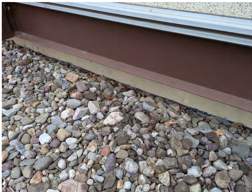
Photograph 16: Concrete waterproof sheeting, observed in the Addition and Tower. Sample numbers 119 and 118, respectively.
